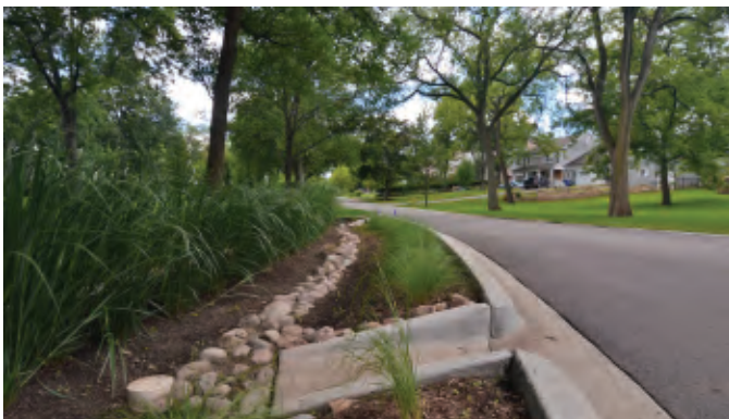
Stormwater runoff from streets needs to be controlled. Trees will slow and intercept stormwater, reducing the burden on stormwater infrastructure.
