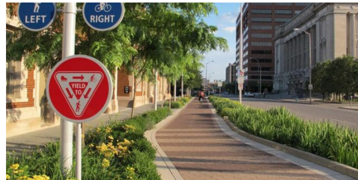
Permeable interlocking concrete pavement and planters manage stormwater runoff, while promoting active transportation. Image Source: Indianapolis Cultural Trail
