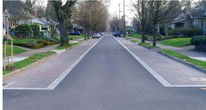
Permeable interlocking concrete pavement infiltrates stormwater and maintains the appearance and functionality of the asphalt street. Image Source: Mutual Materials
