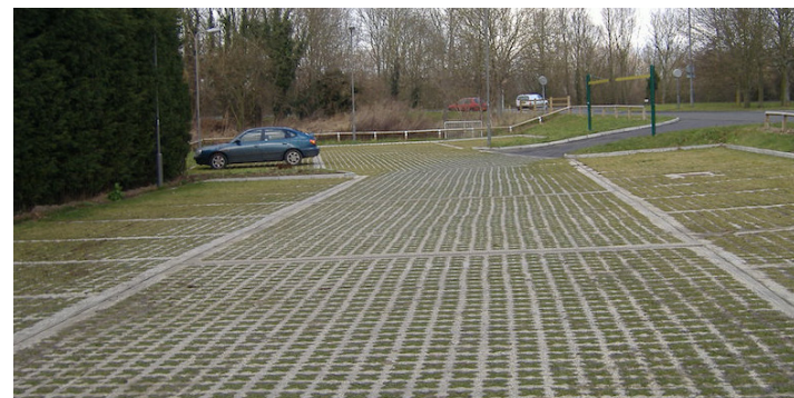
Open grid paving systems filled with grass allow for effective stormwater infiltration and a natural aesthetic. Image Source: GrassConcrete
