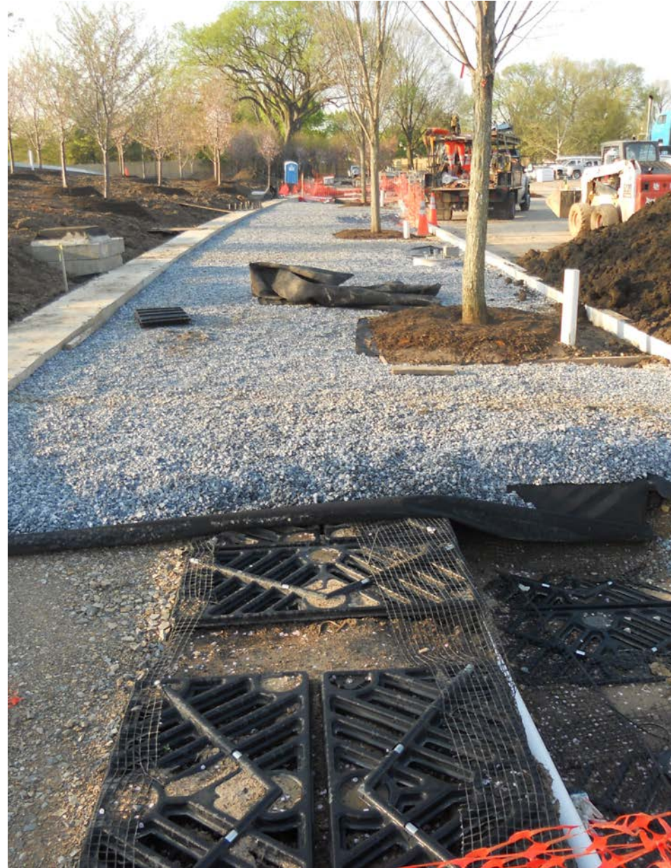
Modular soil cells during installation. Image Source: DeepRoot
