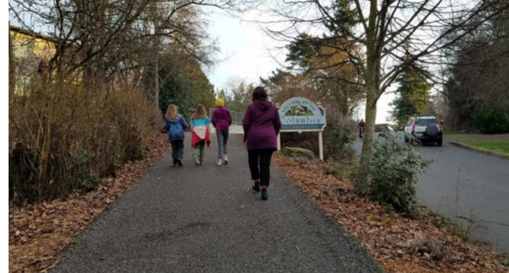
Porous asphalt for a park trail manages stormwater and provides a comfortable and safe user experience. Image Source: City of Bellingham, WA
